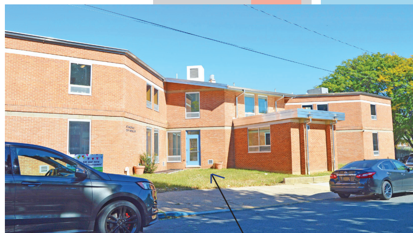
Renovations were completed in October. Outdoor garden and meeting spaces on either side of the community meeting room are still in progress.
